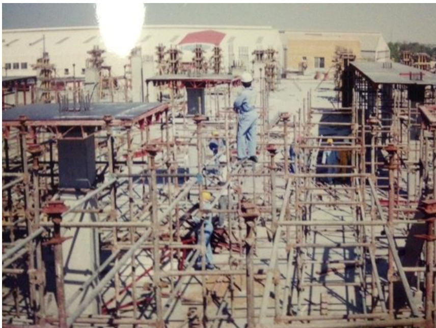
Al Huda Apartment Complex – Dubai Cont'
