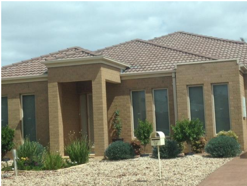
PROJECT 4 - NO: 17, IRONBARK WAY, BROOKFIELD – YEAR 2004/5 (DESIGNED & BUILT)
