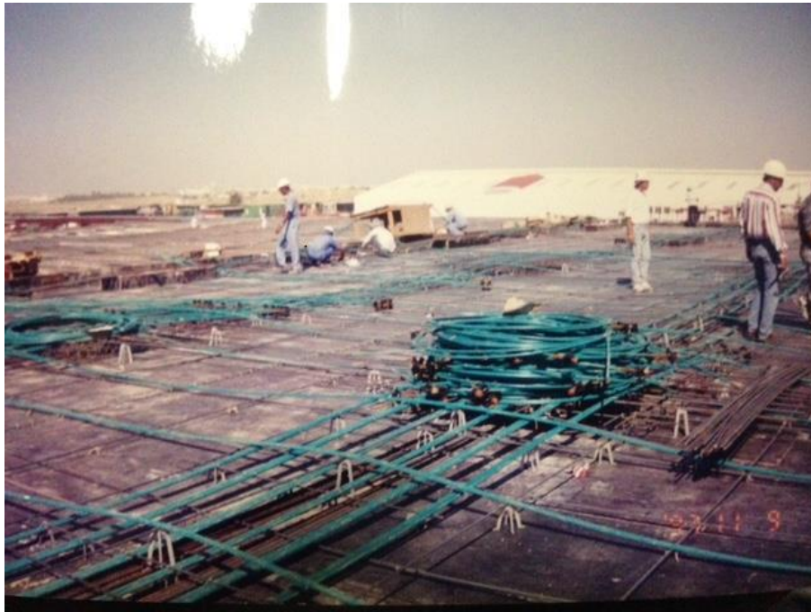
Al Huda Apartment Complex – Dubai Cont'
