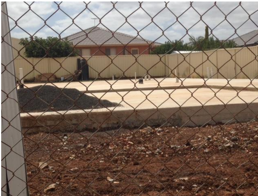
PROJECT 6 - NO: 22-24 THORNHILL STREET, MELTON WEST – YEAR 20015/16 (DESIGNED & BUILT – 4 UNITS) Cont'
