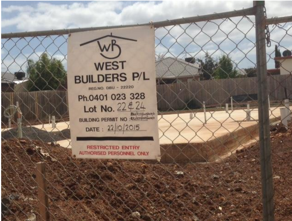
PROJECT 6 - NO: 22-24 THORNHILL STREET, MELTON WEST – YEAR 20015/16 (DESIGNED & BUILT – 4 UNITS)
