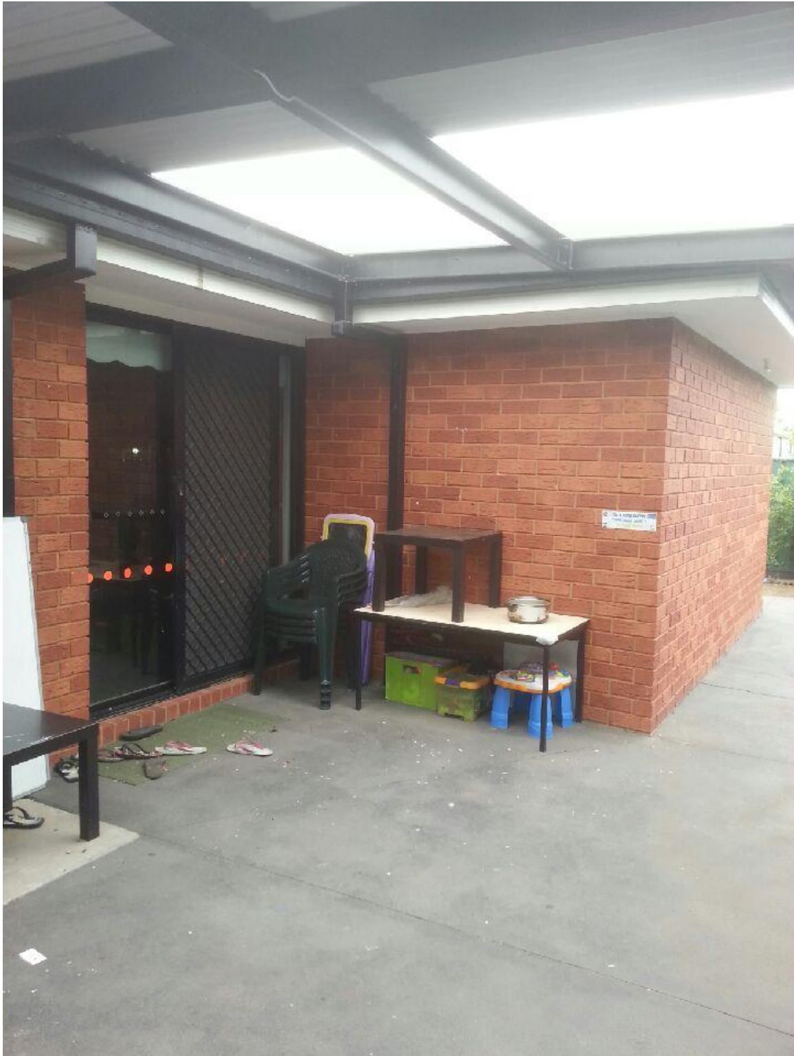
PROJECT 5 - NO: 2, TAURIMA COURT, BURNSIDE – YEAR 2008/9 (DESIGNED & BUILT - EXTENSION)
