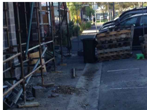
CONCRETE SPOON DRAIN
